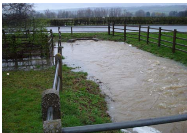
Little Beckford culvert in spate – 03/08 condition
